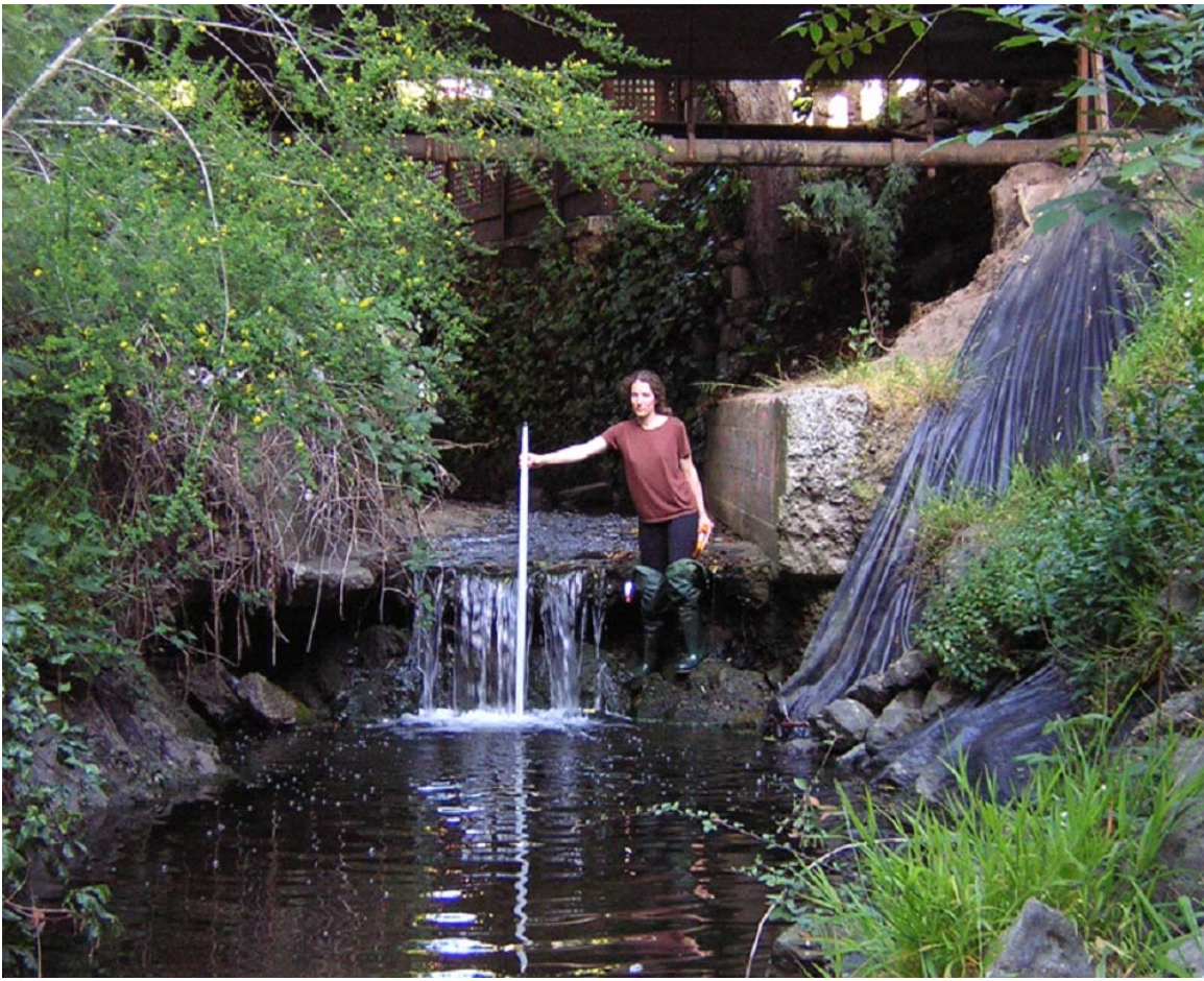
Figure 19. Albina Avenue Bridge crossing and the 4' plunge pool at the outfall.
