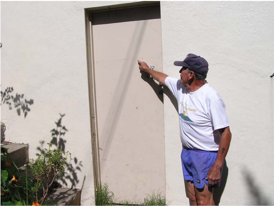
Figure 2. Flooding elevation, as indicated by debris line on a resident's door, experienced upstream of the Cornell Avenue culvert in a January 2004 storm.
